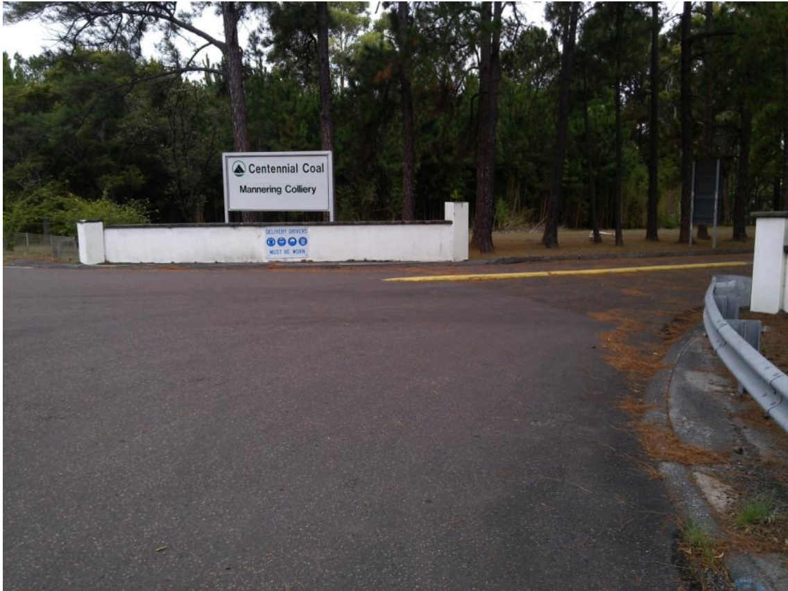
Photograph 9 - Existing Masonry Wall at the site entrance
