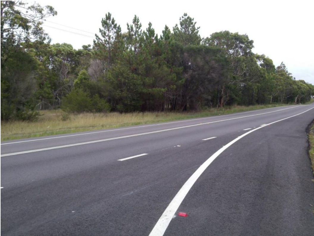
Photograph 6 – Ruttleys Road showing new road pavement at the intersection
