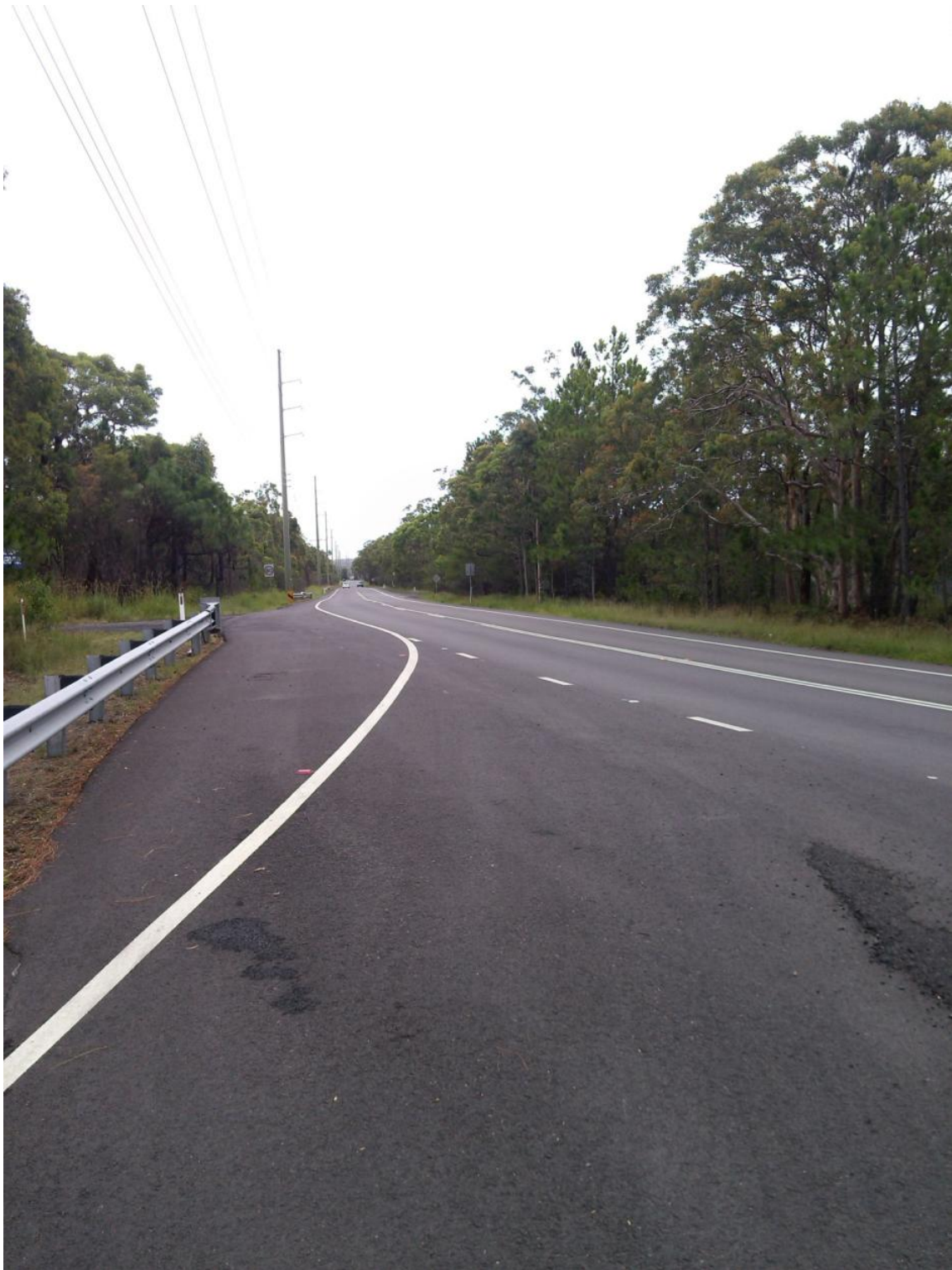
Photograph 5 – Ruttleys Road to the south, showing new linemarking, guardrail and guide posts
